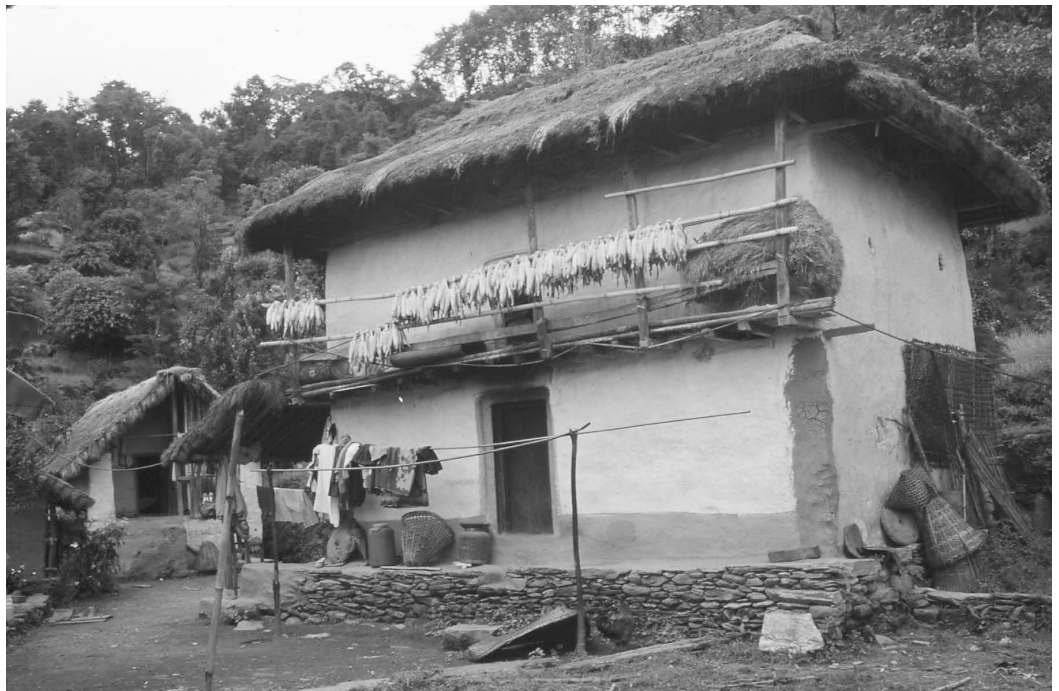
Typical Rai house in Mulgaon Village. Maize is stored outside in the crib, hung below the roof, or inside on the second floor. (Picture P. Gurung)
